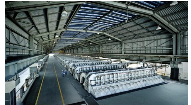
Smelting is the process of extracting Aluminium metal from alumina through electrolytic reduction
